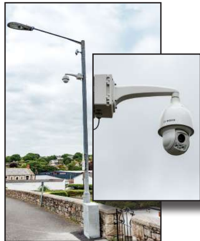
St Austell Town Council owned CCTV in Truro Road
