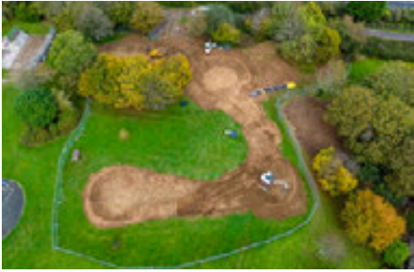
The Meadows Pump Track during construction
