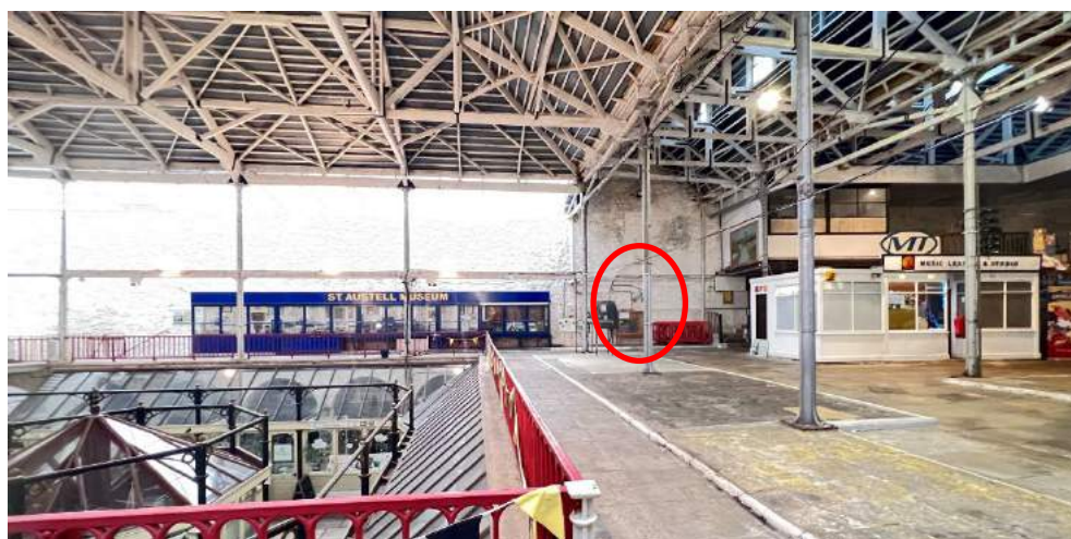
Market House indoors showing the timber roof and cast-iron poles. The arched doorway that has been blocked up is visible at the rear – marked on the photo with a red circle. (Photo from site visit).
