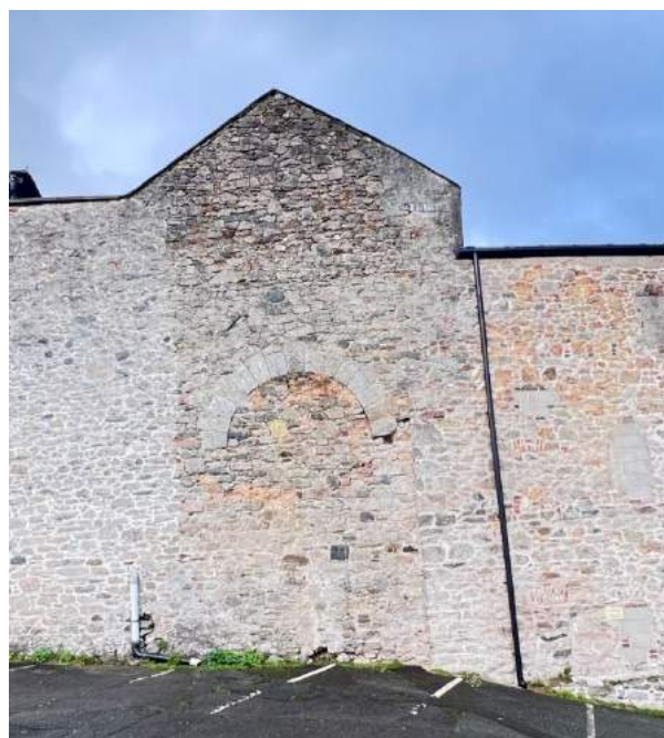
View of Market House from the car park showing the currently blocked up arched doorway. A detail of the variety of stones and blocked up openings which hold a deep connection to the area's rich history can be seen to the right.
