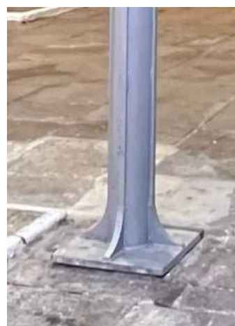
View of Upper Hall taken during site visit demonstrating the seamless integration of the hidden rainwater downpipe system with the structural elements of the building.
