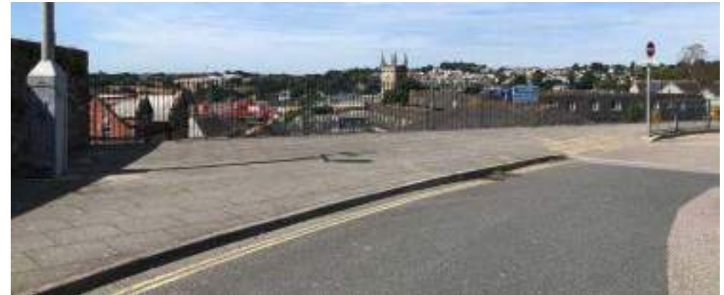
Figure 100. Railway Station town interface
