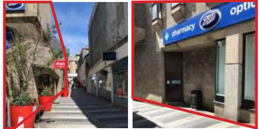
Figure 102. Aylmer Place view of Argos and Boots building
