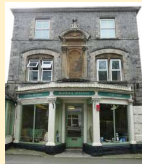
Historic shopfront at 25 Truro road
