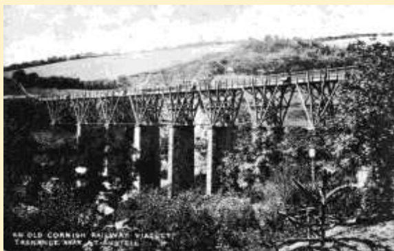
Postcard showing the original Brunel viaduct with its timber trestles supporting the broad-gauge track. The trestles were cheaper to build and designed so timbers could be replaced, but in the long term were much more expensive to maintain
