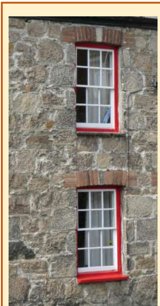
Original small paned windows (without horns) on the cottages on Grove Road.
