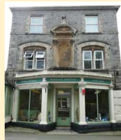
Historic shopfront at 25 Truro road
