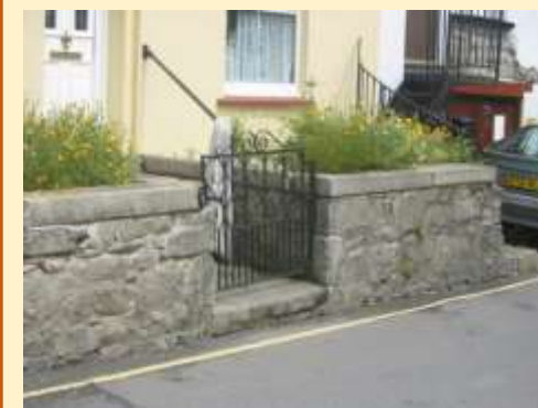
Low stone walls with dressed granite copings bring character and enclosure to the street.
