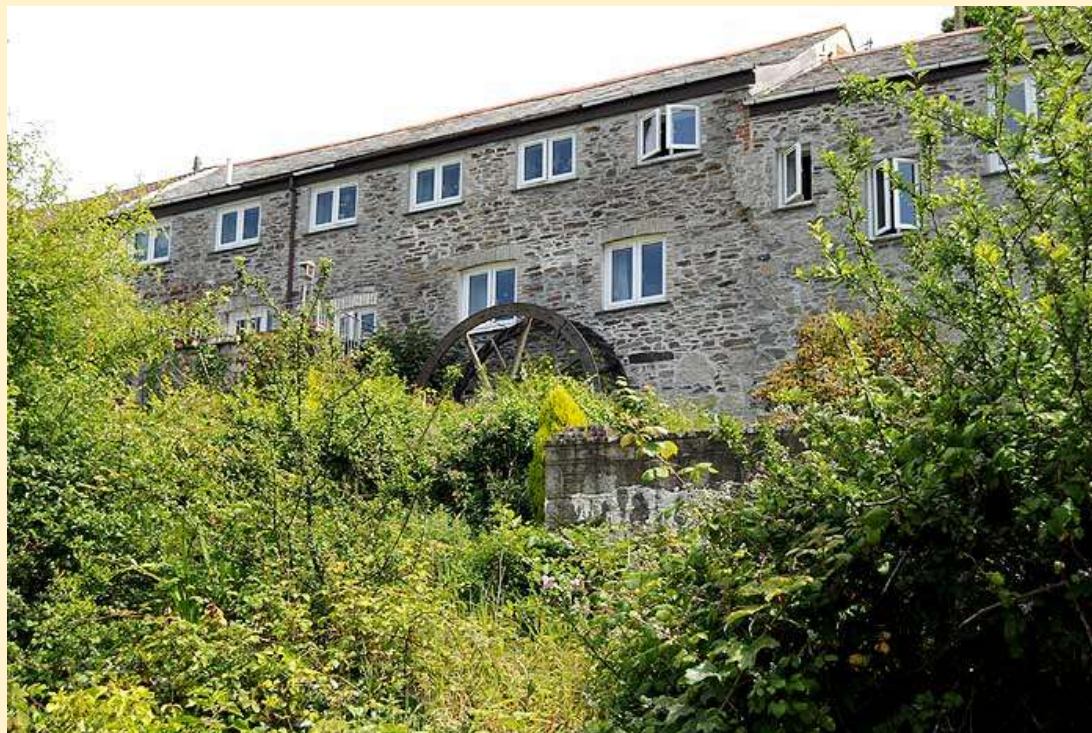
Old mill on Bodmin Road. Located on the route of the leat from Menacuddle, which powered its waterwheel.
