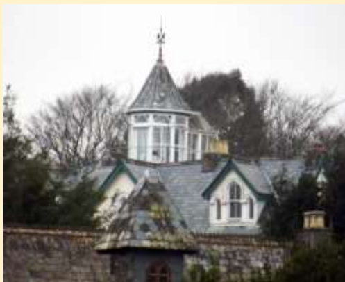
Interesting roofscape in the suburban residential area off Palace Road
